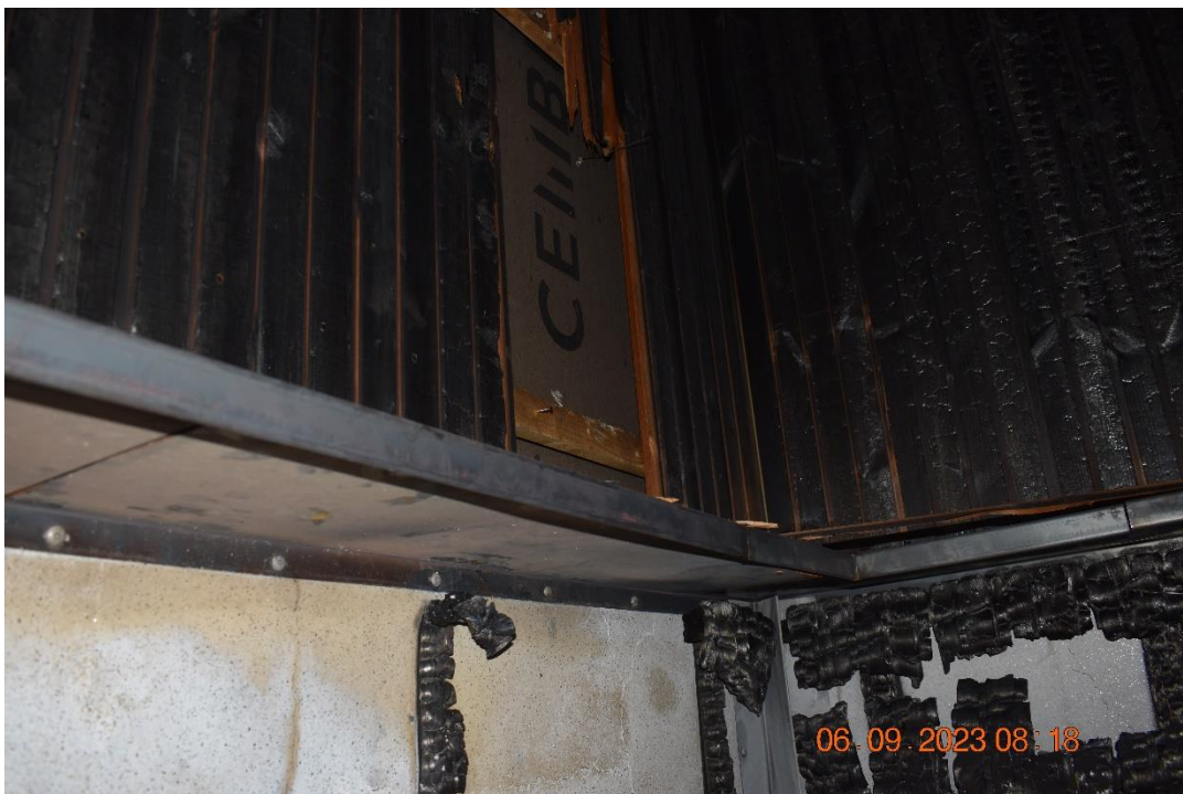
Photo No. 26 Test specimen after the test.
