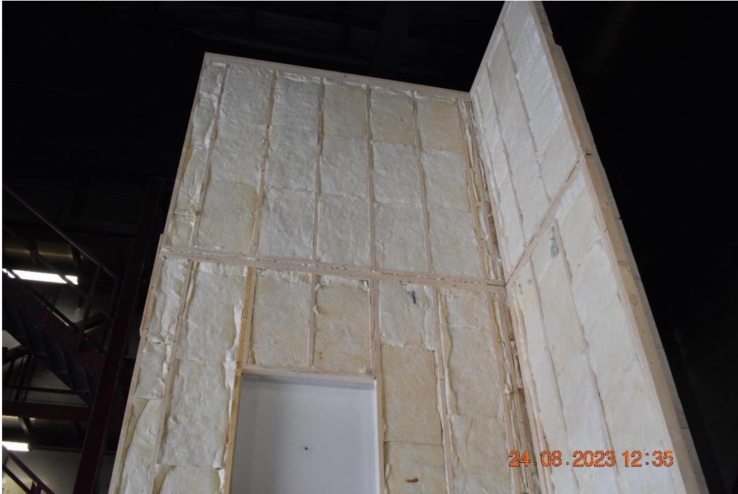
Photo No. 3 Isolation layer applied to the façade.
