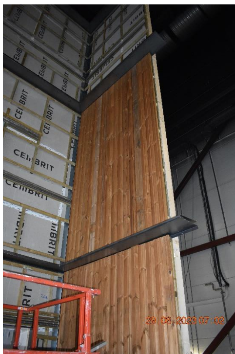
Photo No. 8 Cladding is being mounted.
