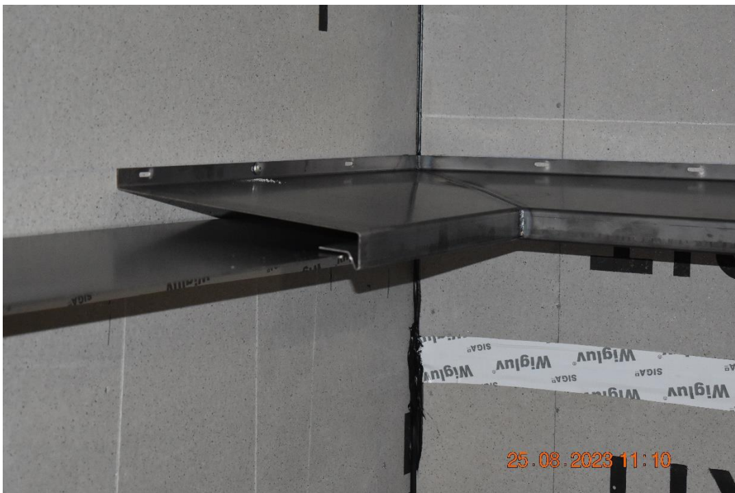
Photo No. 6 Fire breakers are being mounted.
