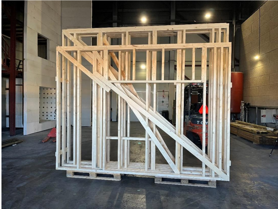
Photo No. 1 Prefabricated cassettes.
