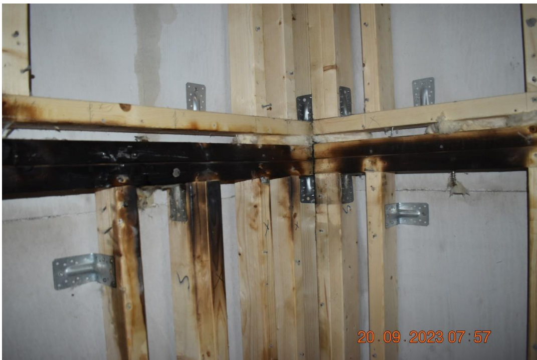
Photo No. 30 Construction wood in the corner at first level.
