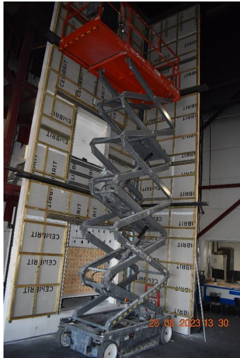
Photo No. 7 Cross formwork and firestop have been mounted.
