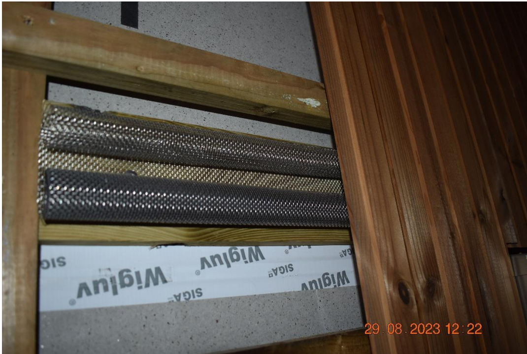
Photo No. 9 Detail of firestop and cladding.
