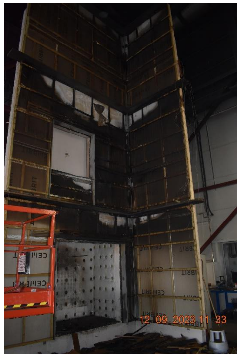
Photo No. 28 All cladding has been removed.
