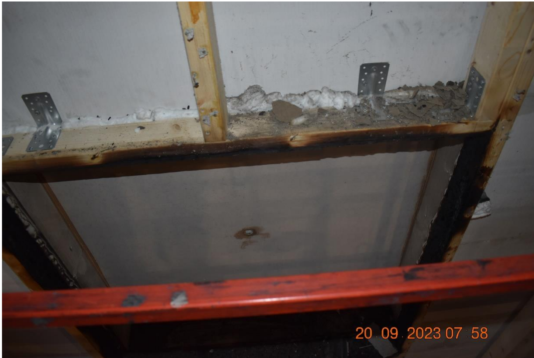
Photo No. 31 Construction wood in at first level.
