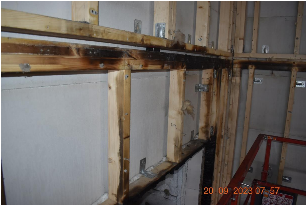
Photo No. 29 Windstopper and insulation has been removed.
