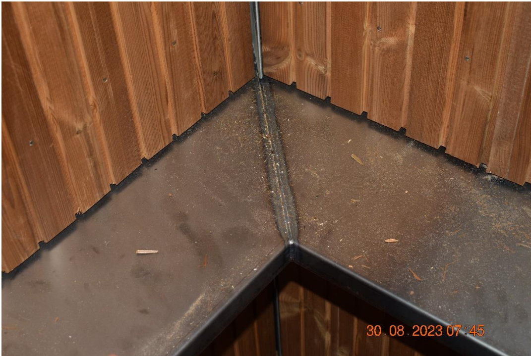
Photo No. 11 Connection between the main façade and wing.
