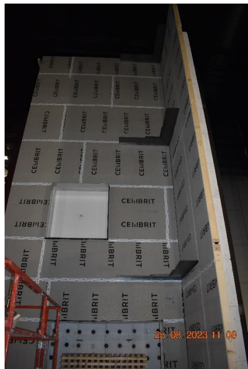
Photo No. 4 Cembrit boards mounted to the prefabricated cassettes.
